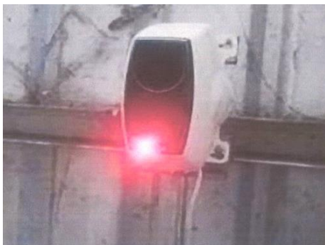
Smoke Beam Detector
